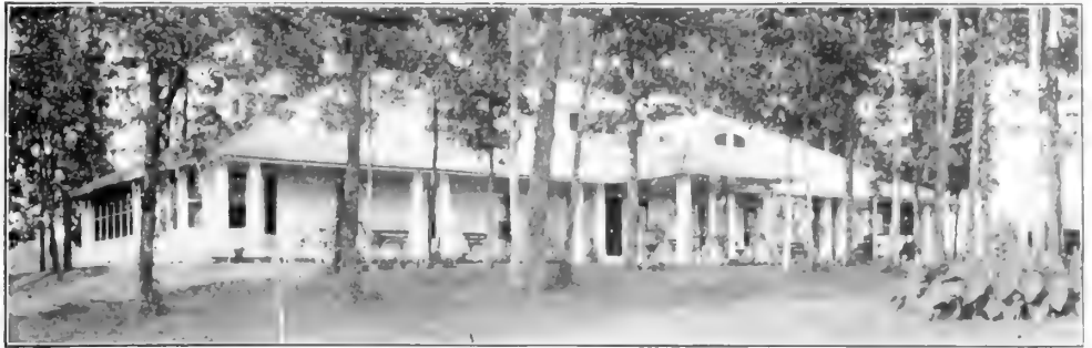
Country Home of Rev. J. Wilbur Chapman, Winona Lake, Ind. Supplied with water by the Kewanee Water Supply System
